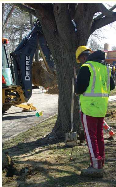
▲ Replace lead service lines in Flint, Michigan.
